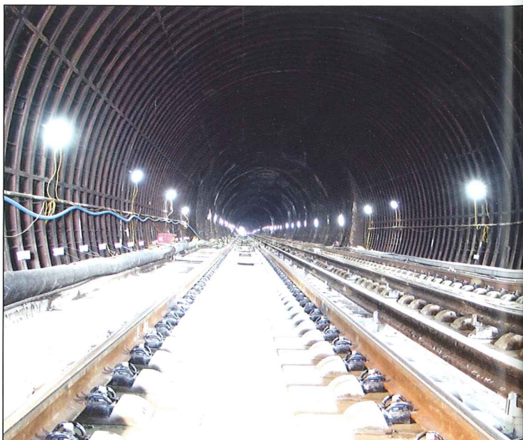
Completed track slab inside the tunnel prior to final cleaning.
