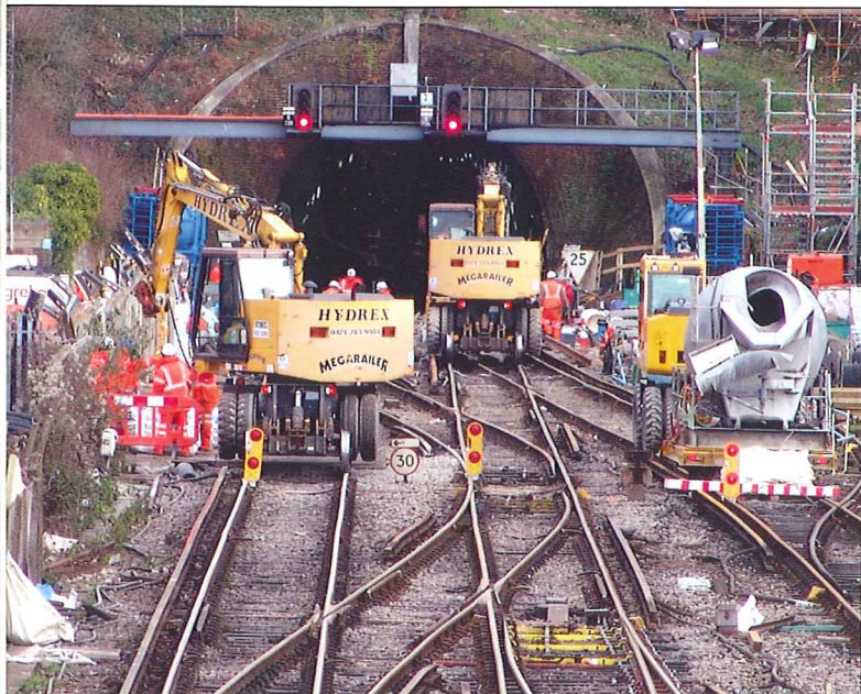
Southampton Central Station throat showing worksite limits.
