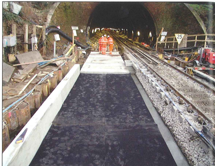
Ballast trough and transition slab prior to track installation.
