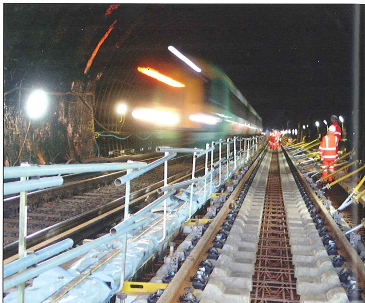
Down Line construction with train passing on Up Line.
